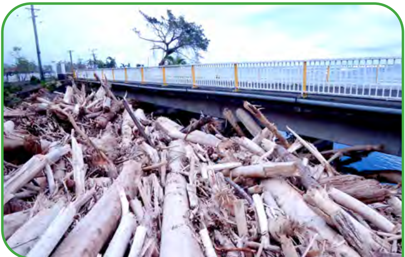
Shallow rooted Albizia causing blockage to river ways affecting infrastructure in Samoa during Cyclone Evan.
